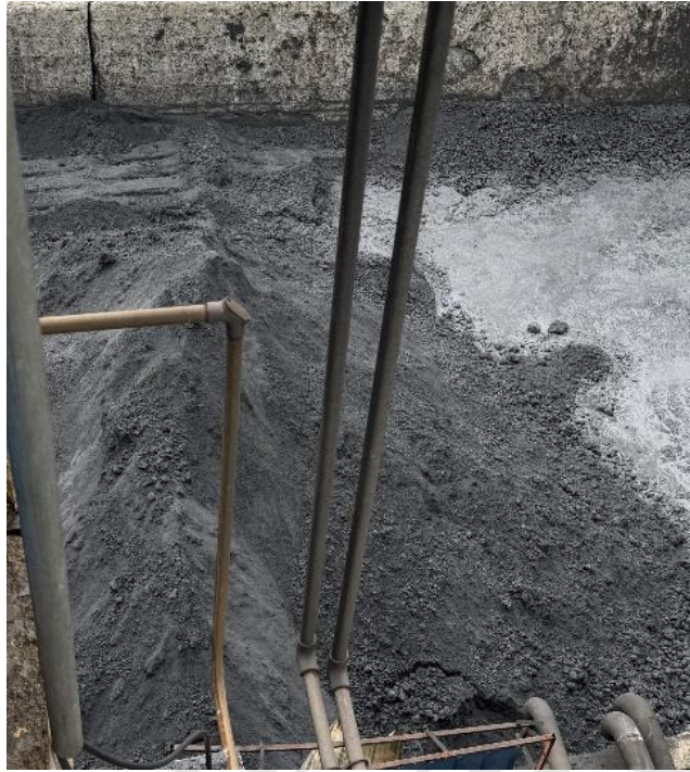
Figure 3 Coke pit without Crusher
