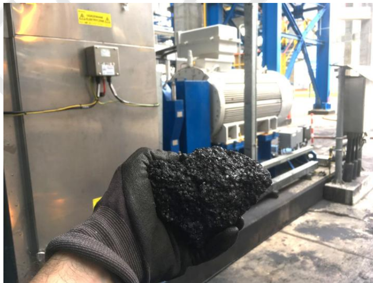
Figure 4 Coke after Crusher with ECHO
